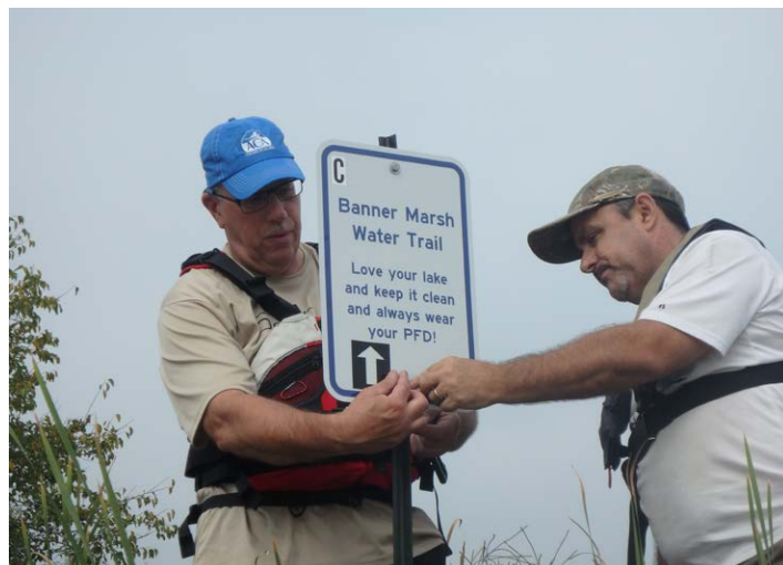
Two ACA-certified canoe instructors, Jeff Fitch and Dave Watts, installed signs for the newest watertrail in Illinois in late September.
