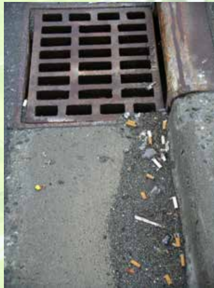
Cigarette butts wash down a storm drain on Tudor Road in Anchorage. C. Northon photo
